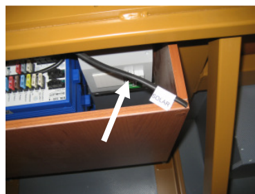
Pre-wiring at battery charger
