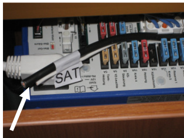
Pre-wiring at battery charger
