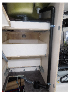
Screwed siphon of sink
