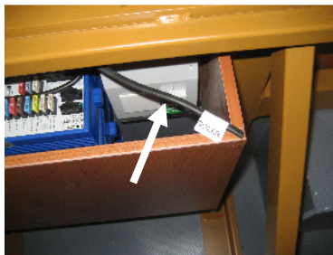
Pre-wiring at battery charger
