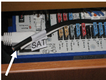
Pre-wiring at battery charger
